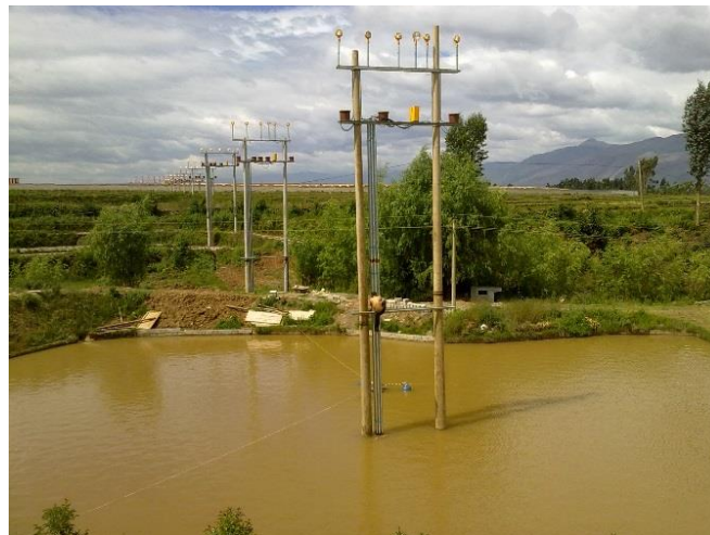
Figure 3.9 Installation Field Figure of Elevated Mast
